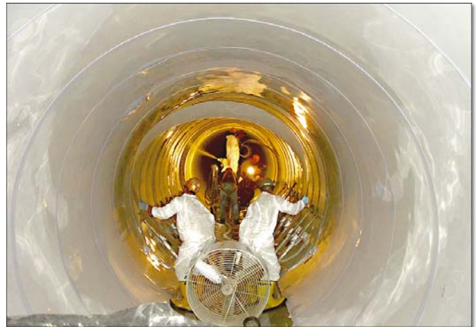
Above: The Linabond Structural Polymer Pipeline Spray System™ is ideal for rehabilitation of pipelines and brick sewers. Flexible PVC is used over (cross-linked into) the structural polymer in this system to repair and line the pipeline.
