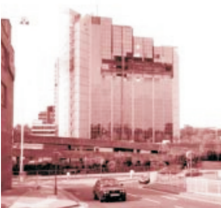
The steel frame at the Churchill Plaza, Basingstoke is protected with Mandolite CP2.
