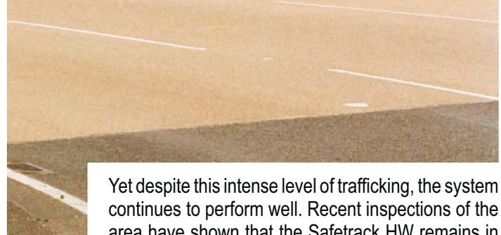
Yet despite this intense level of trafficking, the system continues to perform well. Recent inspections of the area have shown that the Safetrack HW remains in good condition and continues to provide excellent skid resistance. Whilst Safetrack HW may not have initially been the lowest first-cost option, its performance far surpasses that of traditional thermoplastic systems, which if used in this location would probably have been needed to be replaced three times already.
